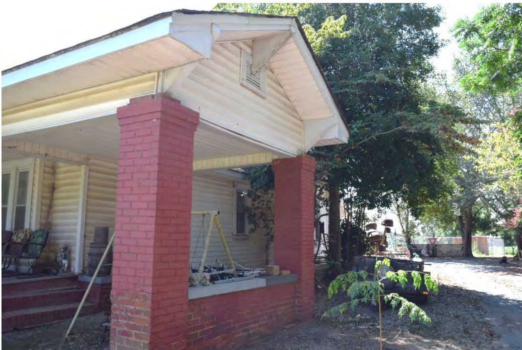
Braswell House, Side (West) Elevation and Porte Cochere, Looking East.
