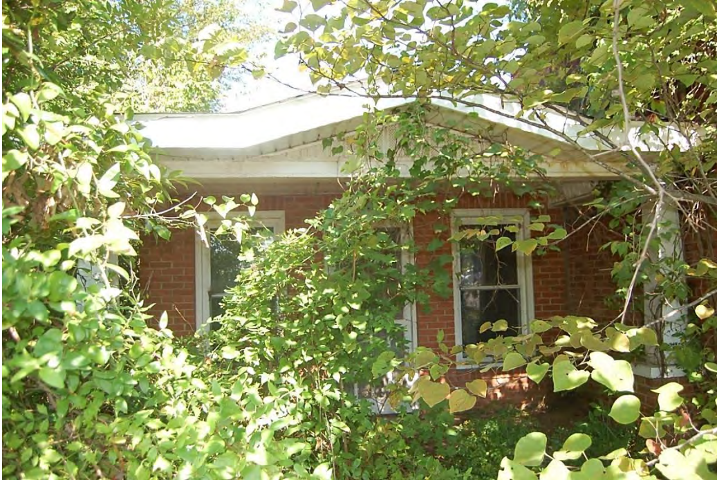
Helms-Kiker Store, Residential Wing, Façade (South Elevation), Looking North.
