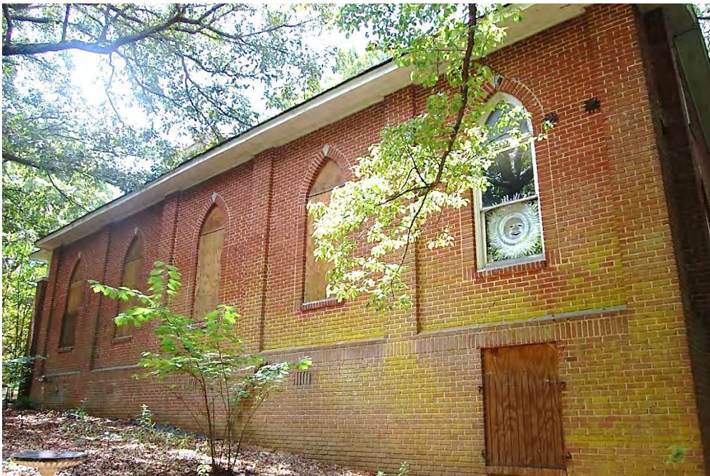
Tabernacle Presbyterian Church, (Side) East Elevation, Looking Southwest.
