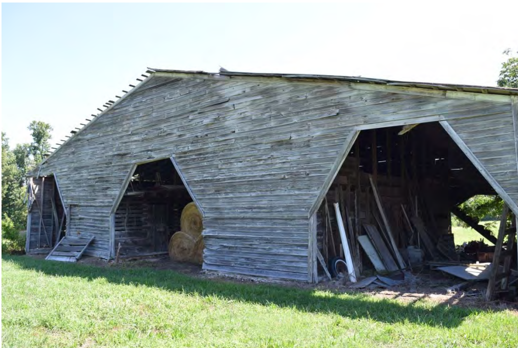
Clonnie Moore House No. 2, Barn, Looking Northeast.
