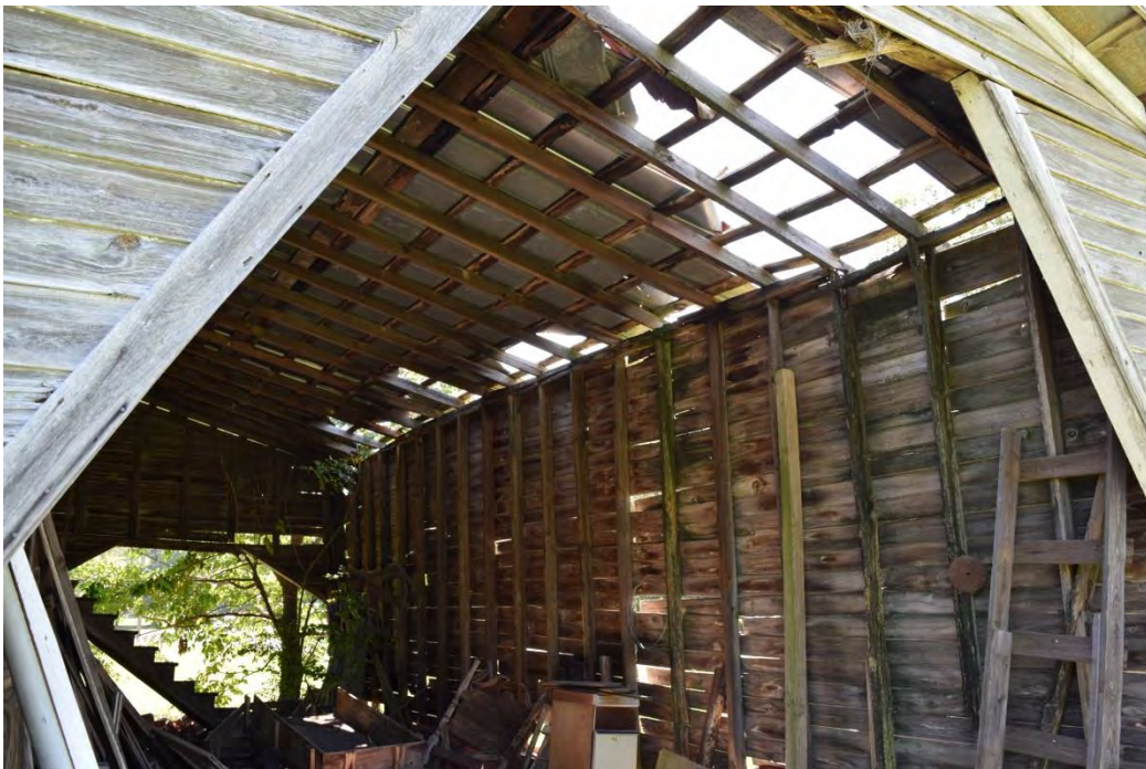
Clonnie Moore House No. 2, Barn, Interior, South Crib, Looking Southeast.
