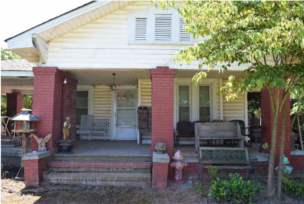
Braswell House, Façade, Looking South.
