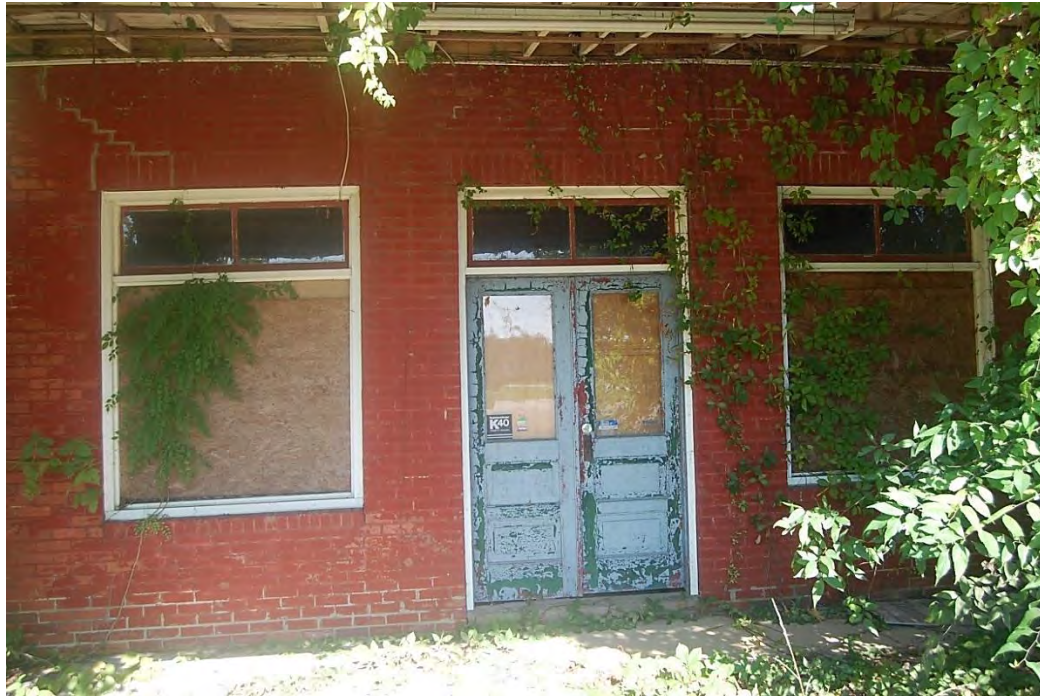
Helms-Kiker Store, Facade, Looking West.
