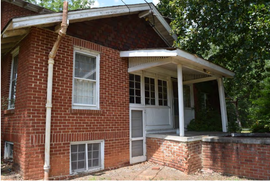
Clonnie Moore House No. 2, Side (East) Wing and Utility Room, Looking Northeast.
