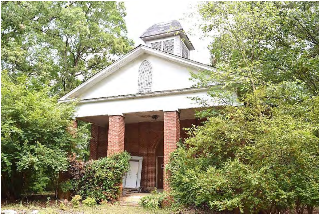
Tabernacle Presbyterian Church, Façade, Looking Northwest.
