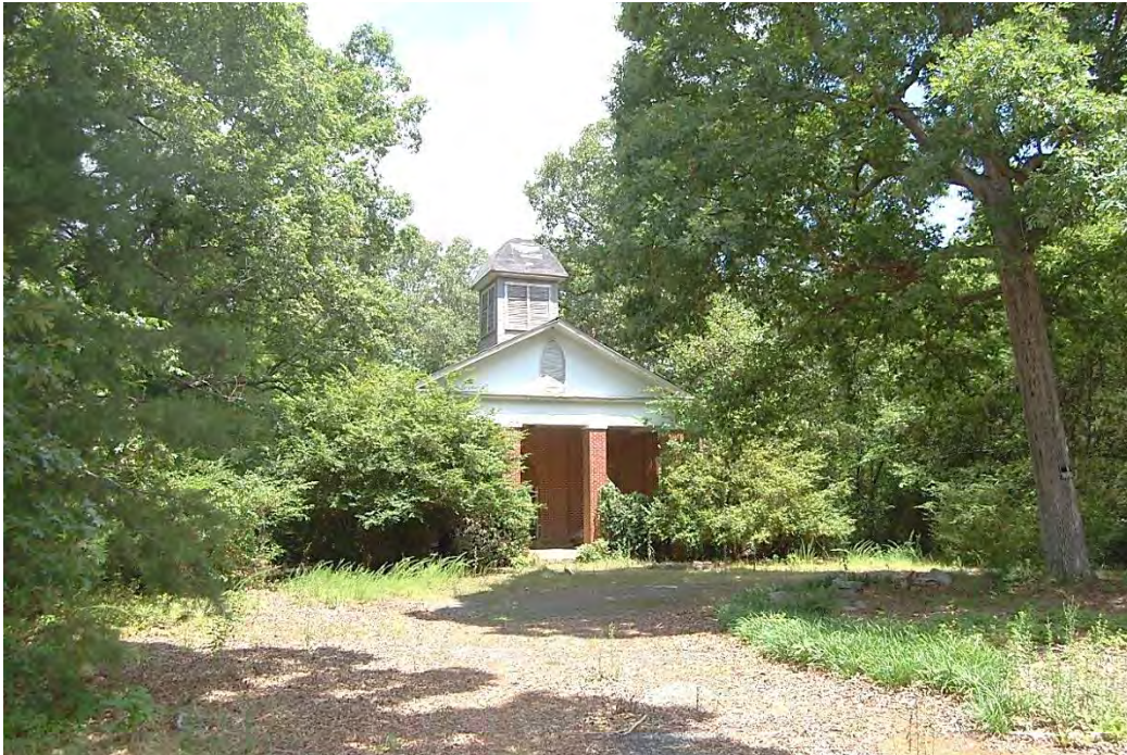
Tabernacle Presbyterian Church, Overall View of Church and Setting, Looking North From NC 205.
