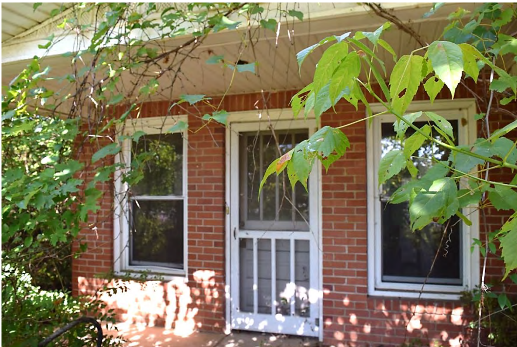
Helms-Kiker Store, Residential Wing, Façade, Looking North.
