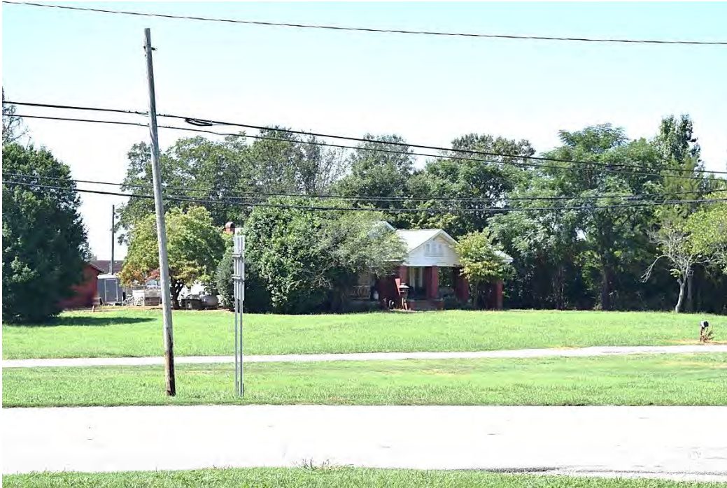
Braswell House, Overall View of House and Setting, Looking Southwest From Clonnie Moore House No. 2.
