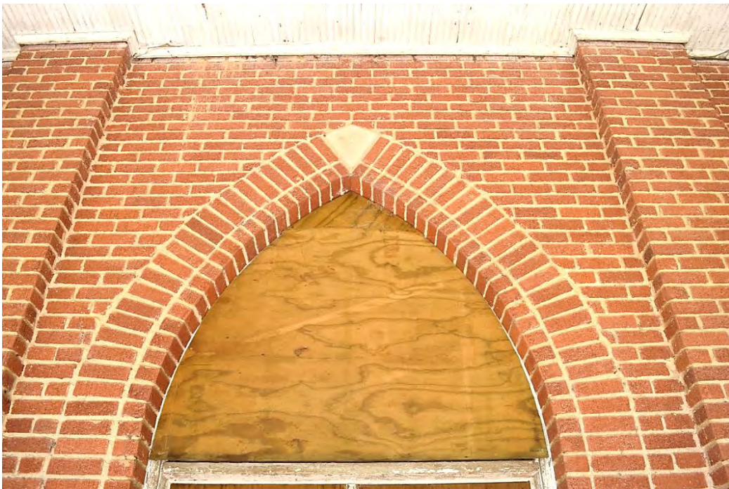
Tabernacle Presbyterian Church, Entrance, Pointed-Arch Transom.
