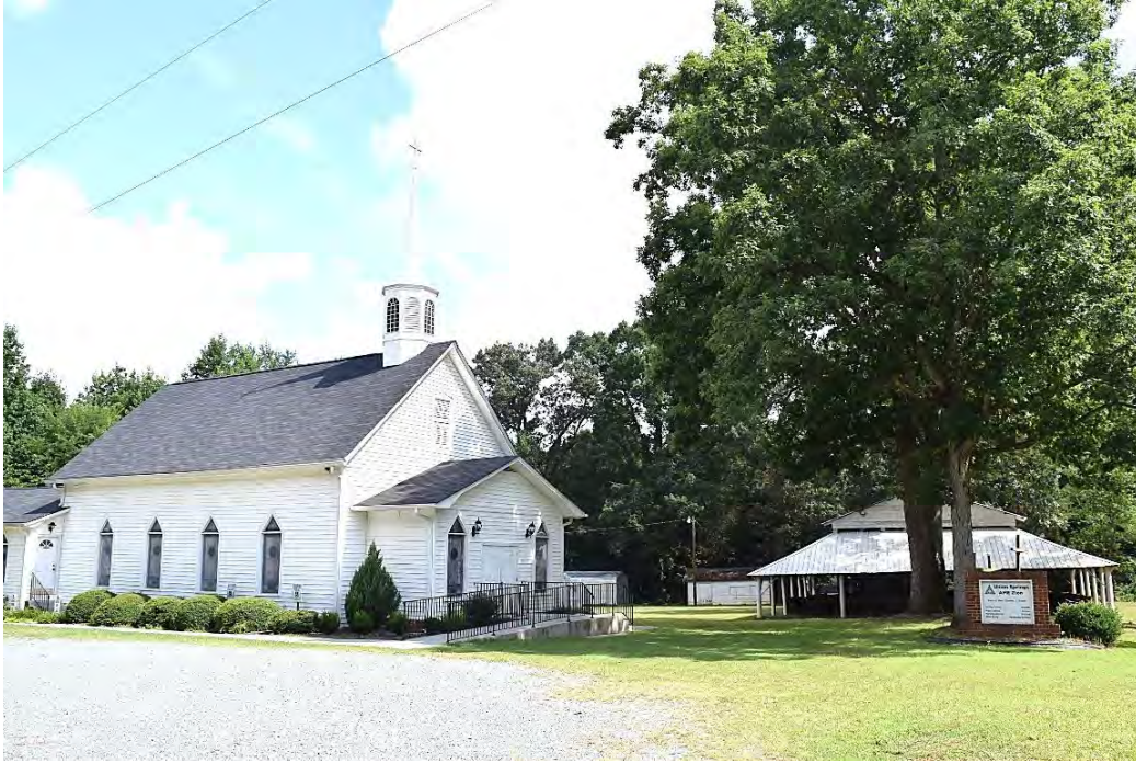
Union Springs AME Zion Church and Arbor, 1877, 1921, 4003 Morgan Mill Road, Monroe Vicinity.
