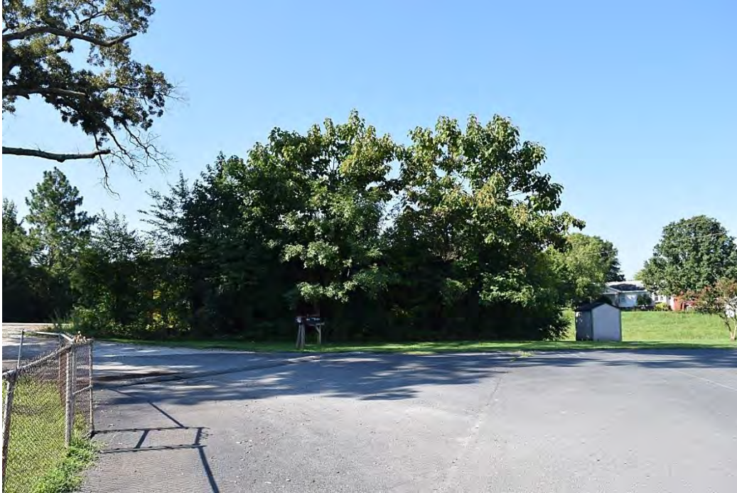
Helms-Kiker Store, Dense Overgrowth along Side (North) and West (Rear) Elevations, Looking South Towards NC 205.
