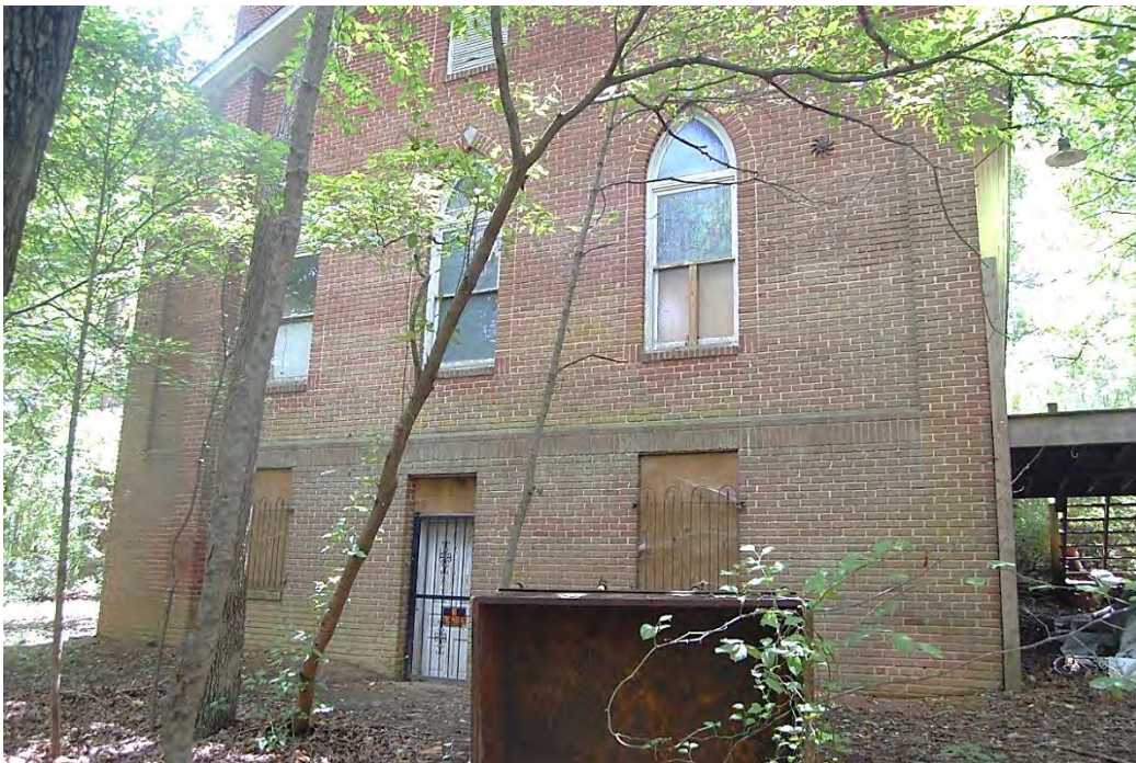
Tabernacle Presbyterian Church, Rear (North) Elevation, Looking South.
