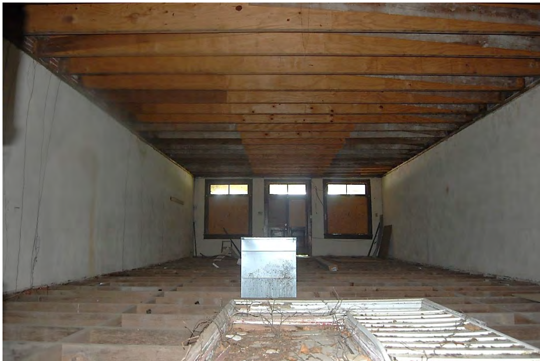
Helms-Kiker Store, Interior, Looking East From Rear (West) Elevation Towards Front.
