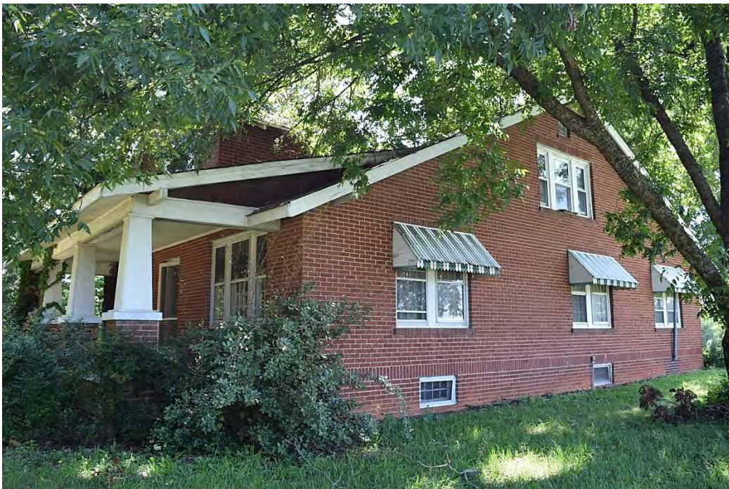
Clonnie Moore House No. 2, Side (West) Elevation, Looking Southeast.
