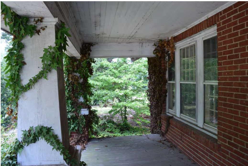
Clonnie Moore House No. 2, Porch and Window Detail, Looking East.
