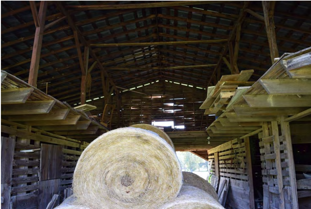
Clonnie Moore House No. 2, Barn, Interior, Center Passage, Looking East.
